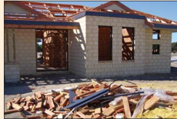
Poor management of untreated pinewood waste (such as off-cuts pictured here) may be putting our homes at risk
