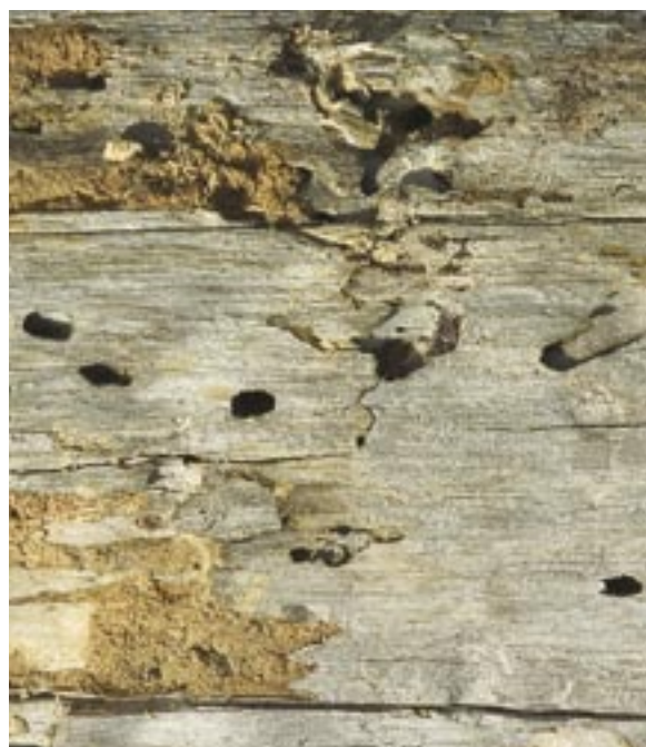
Damage caused by the European House Borer
